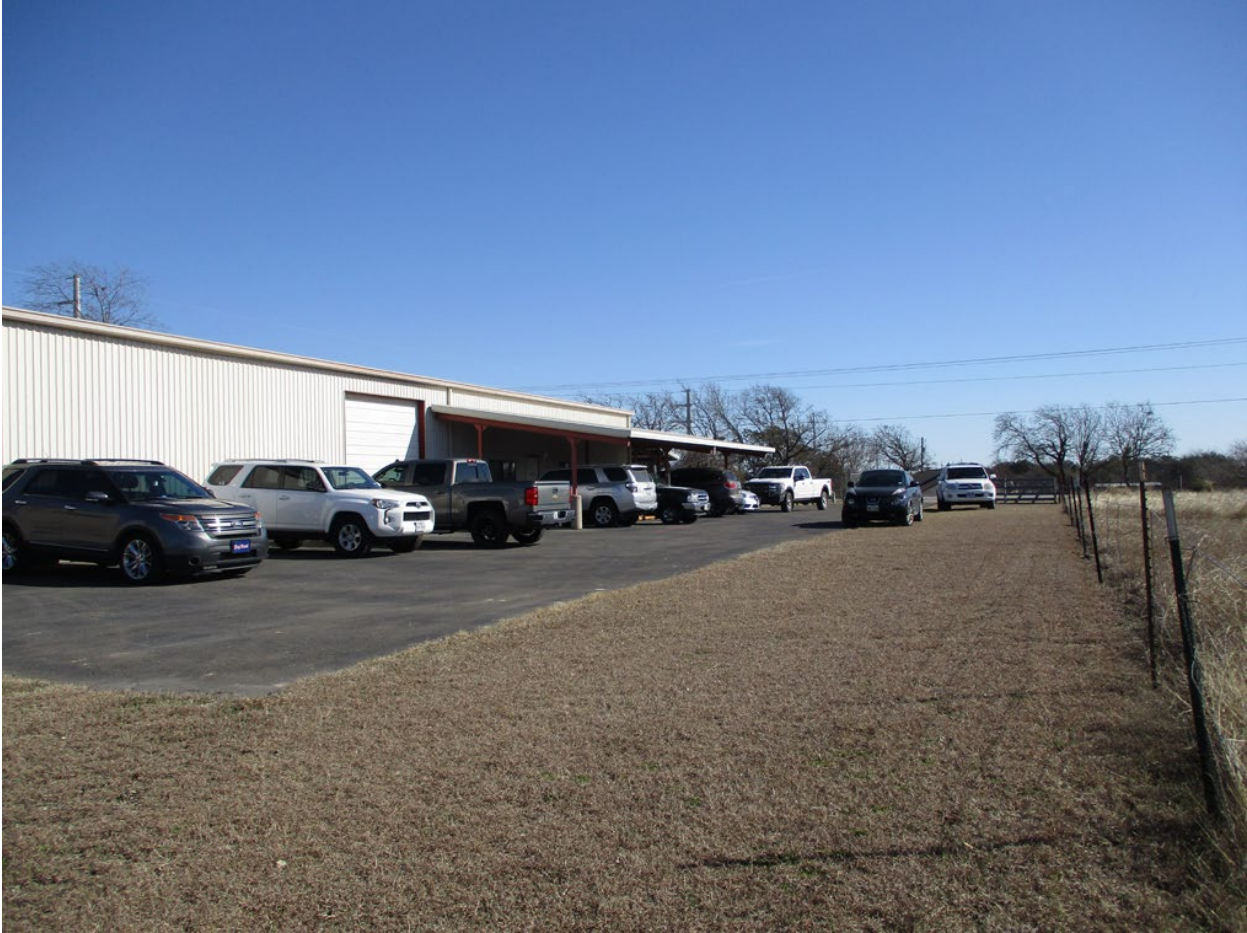
Southern Elevation of of Office/Warehouse Building:
